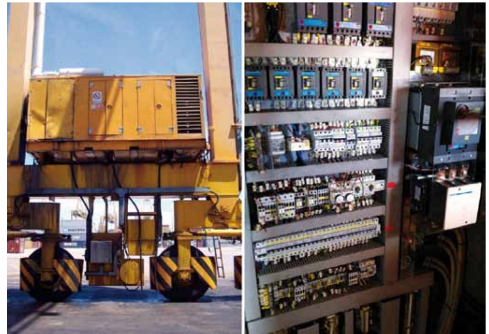
Figure 25. Example of Gen-Set Room and Electrical Control System
