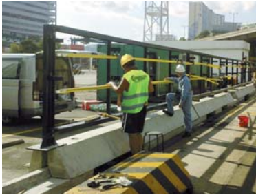
Standardized concrete base and steel framing to mount conductor bars
